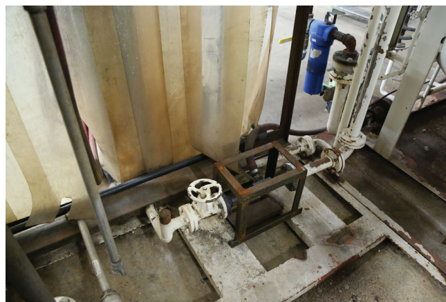
Figure 3: Eductor used for moving IX resin.
